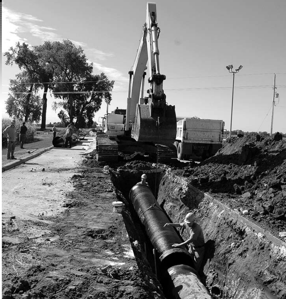
At the Fremont job, Penro crews are laying 2.5 miles of 30-inch water main to bring water from a well field into the city's treatment plant.
